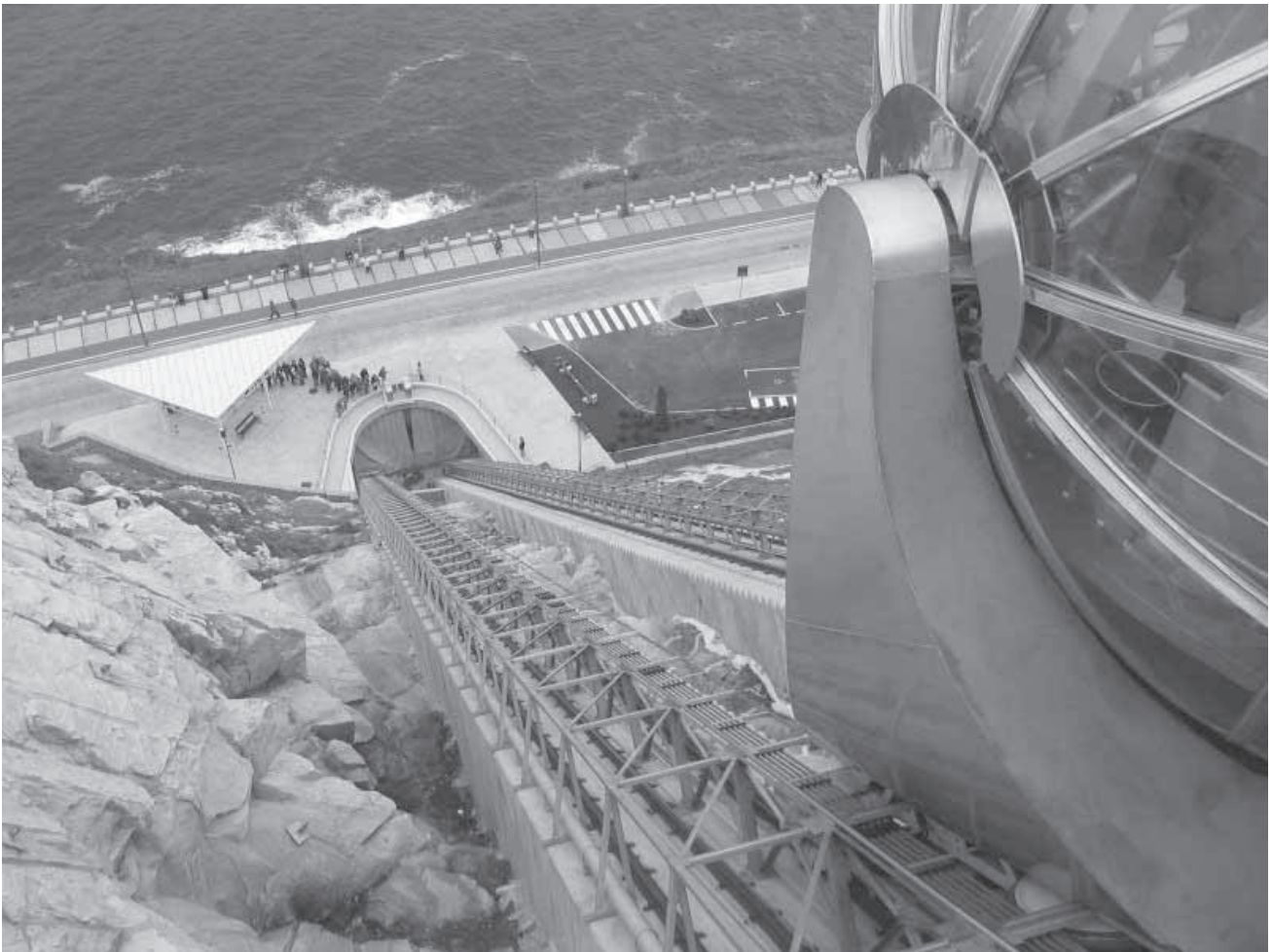
Inclined elevator A Coruña
